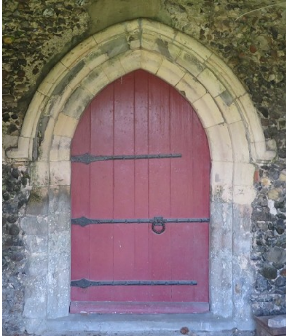
Figure 35 West door into tower
