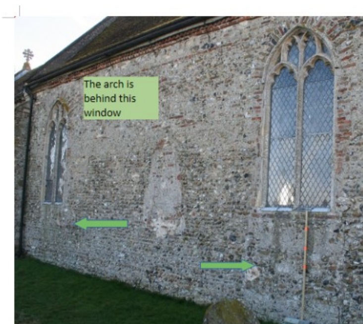
Figure 23 exterior view of where tomb arch lies
