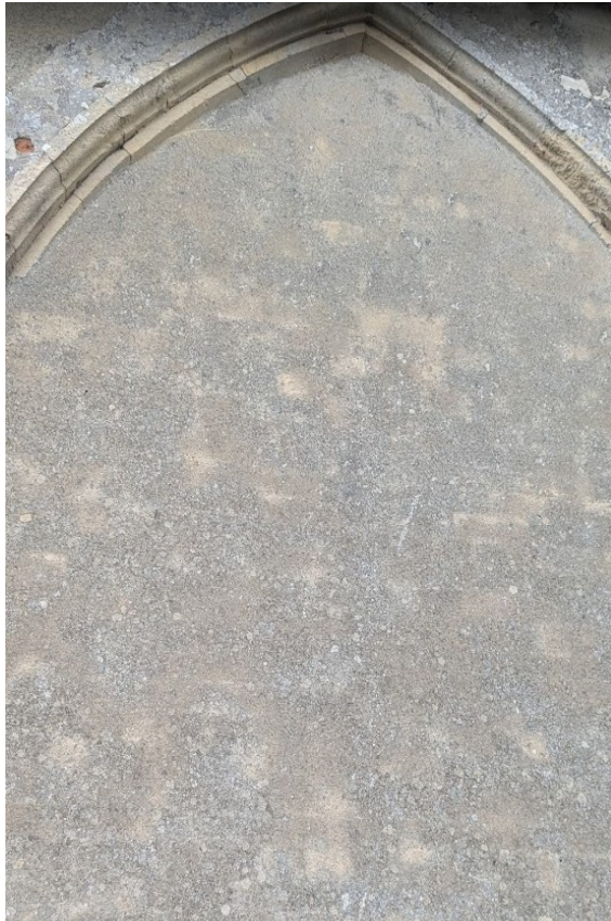
Figure 14 blocked north chancel window
