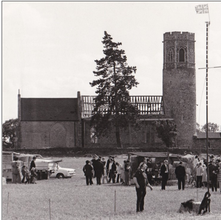
Figure 15 re-roofing of nave in 1974
