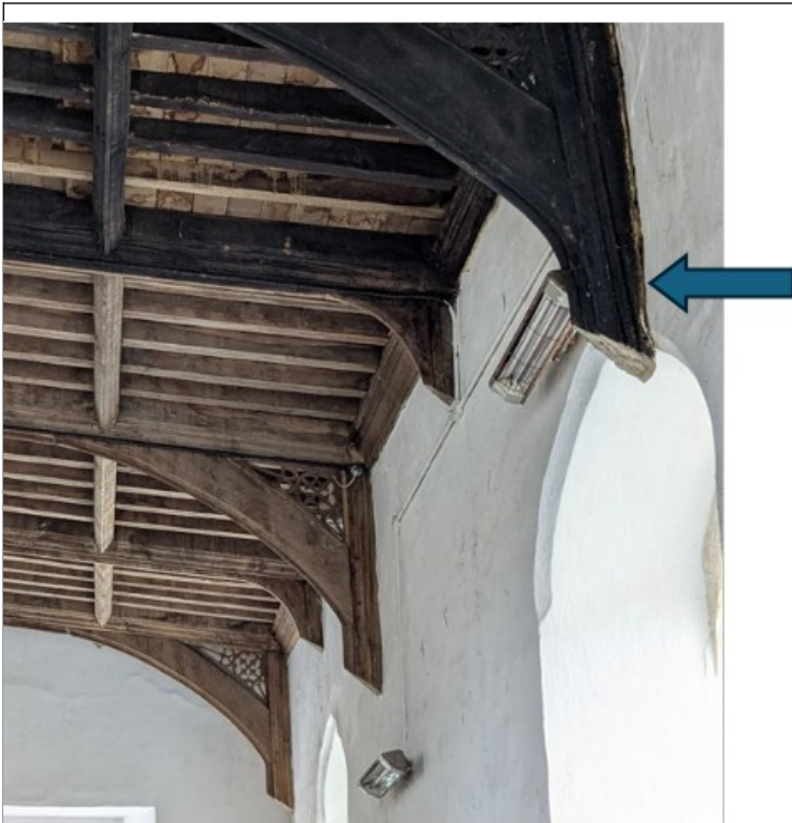
Figure 29 South Aisle roof structure
