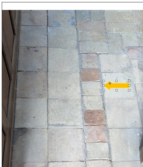
Figure 21 eastern floor of aisle
